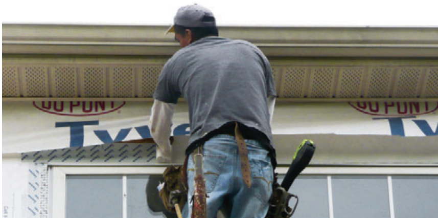
Figure 4. A worker lifts the StuccoWrap along the top of the wall to tape the top fin of the window to the sheathing (above). Metal lath is installed on top of Grade D paper in preparation for stucco (left).
