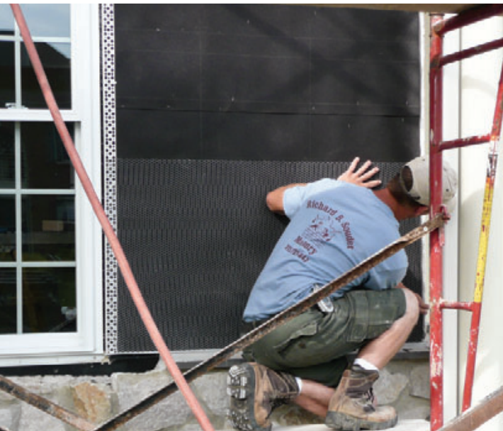
Figure 4. A worker lifts the StuccoWrap along the top of the wall to tape the top fin of the window to the sheathing (above). Metal lath is installed on top of Grade D paper in preparation for stucco (left).
